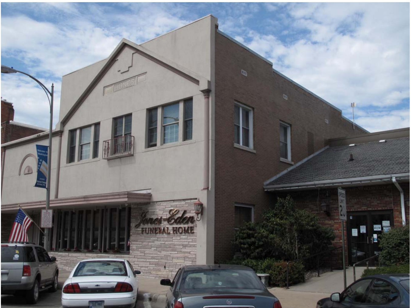
Photograph 92-00536-001 - South and east elevations, looking northwest (McCarley, September 20, 2011).
