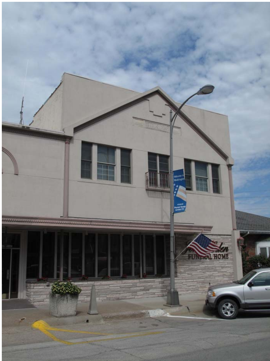
Photograph 92-00536-002 - South elevation, looking northeast (McCarley, September 20, 2011).
