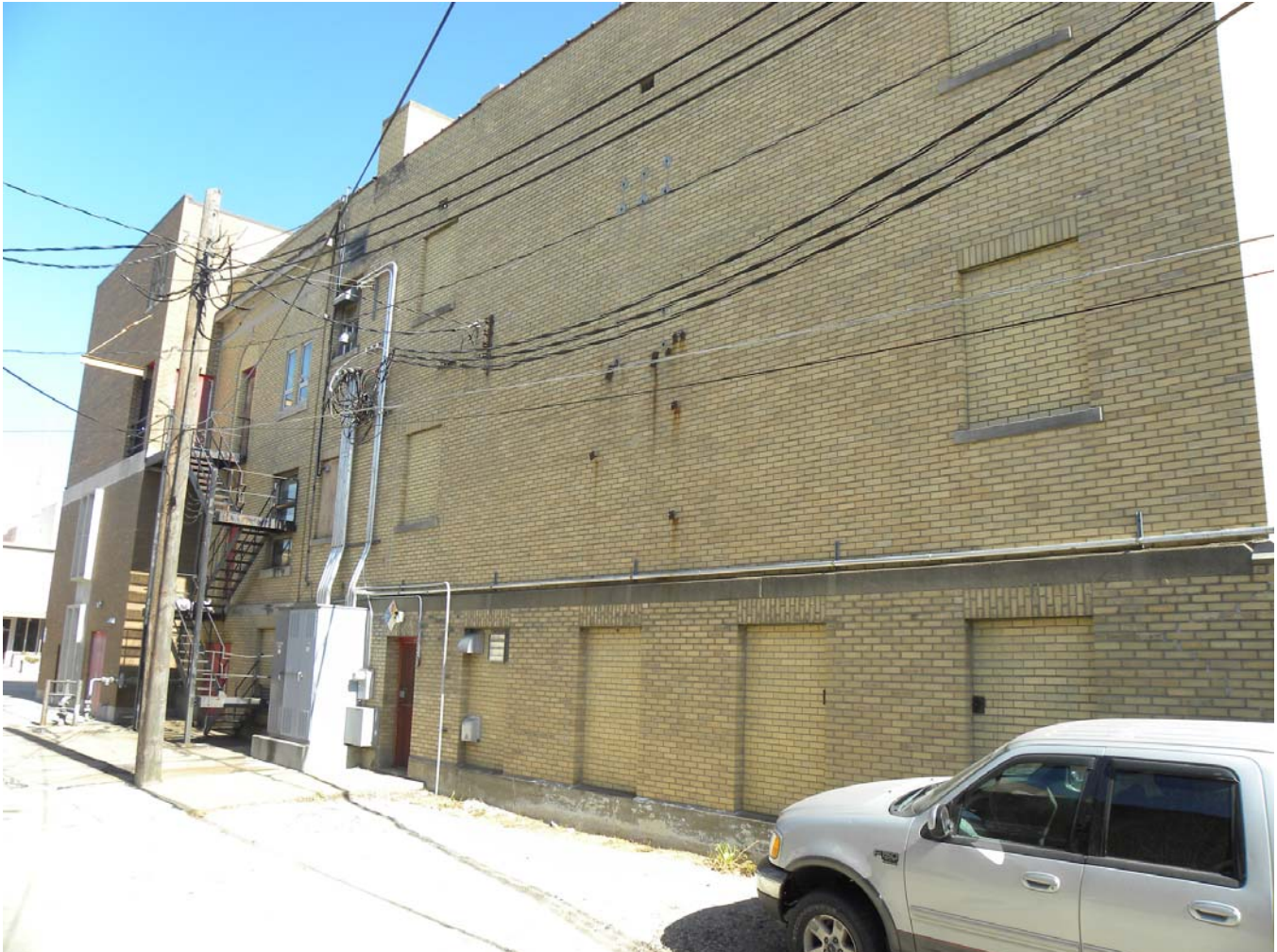
Photograph 92-00537-004 - West elevation, looking northeast (Patterson, October 7, 2012).
