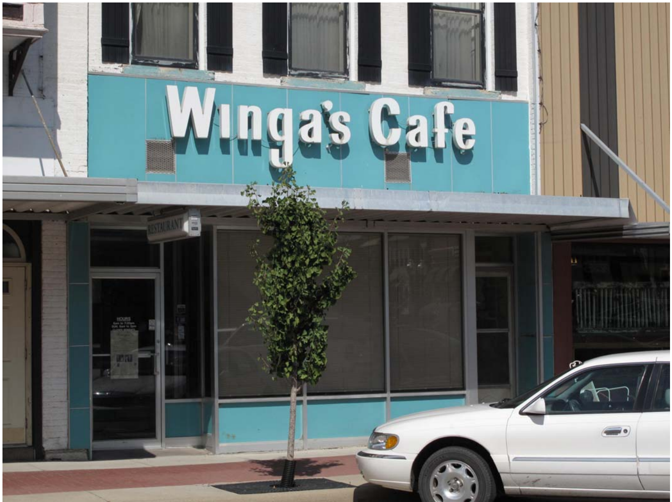
Photograph 92-00539-002 - Detail of storefront, looking north-northeast (McCarley, September 20, 2011).
