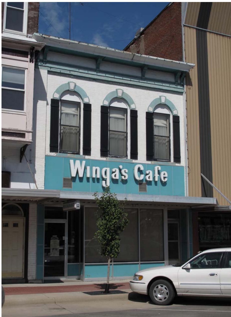
Photograph 92-00539-001 - South elevation, looking northeast (McCarley, September 20, 2011).
