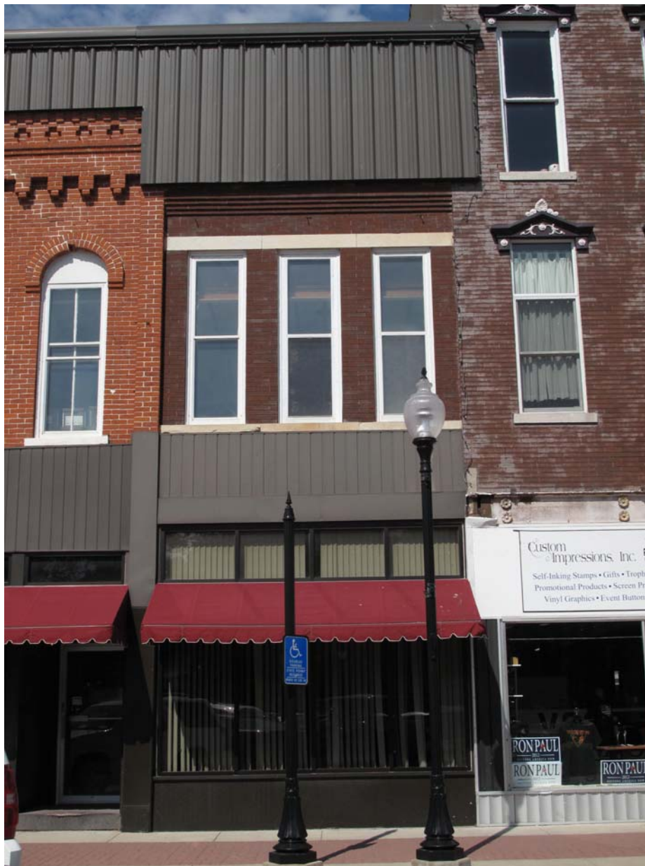
Photograph 92-00541-001 - South elevation, looking north (McCarley, September 20, 2011)
