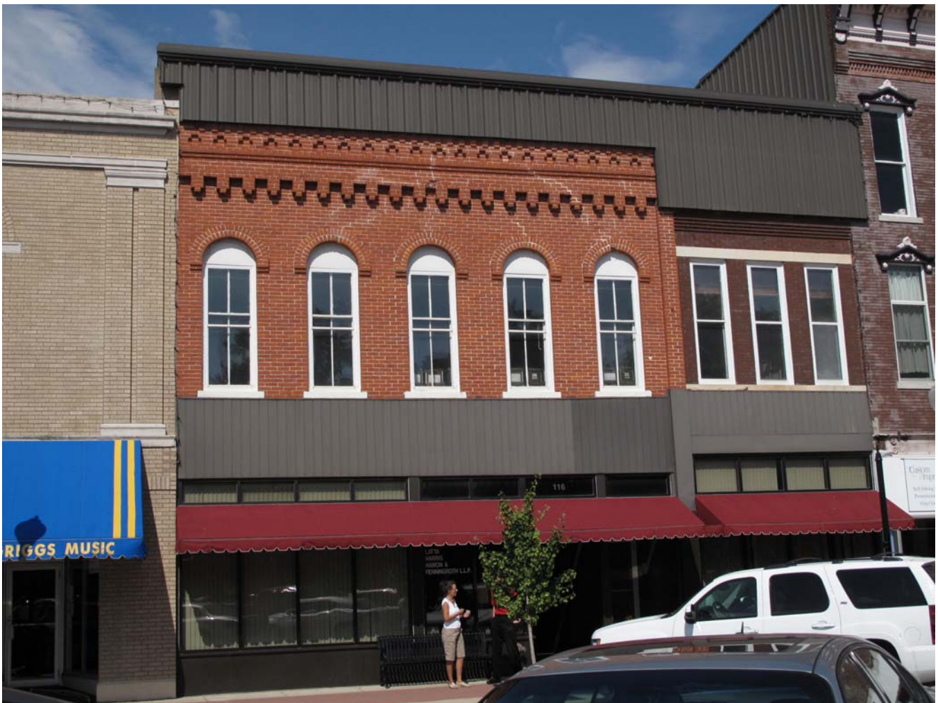
Photograph 92-00542-001 - South elevation, looking north (McCarley, September 20, 2011)
