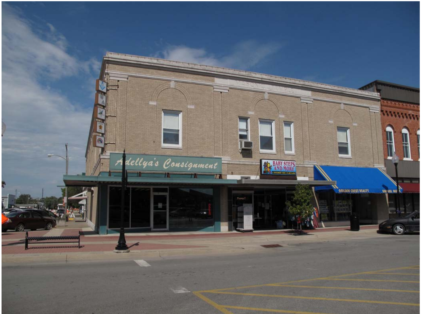
Photograph 92-00543-002 - South elevation, looking north (McCarley, September 20, 2011)
