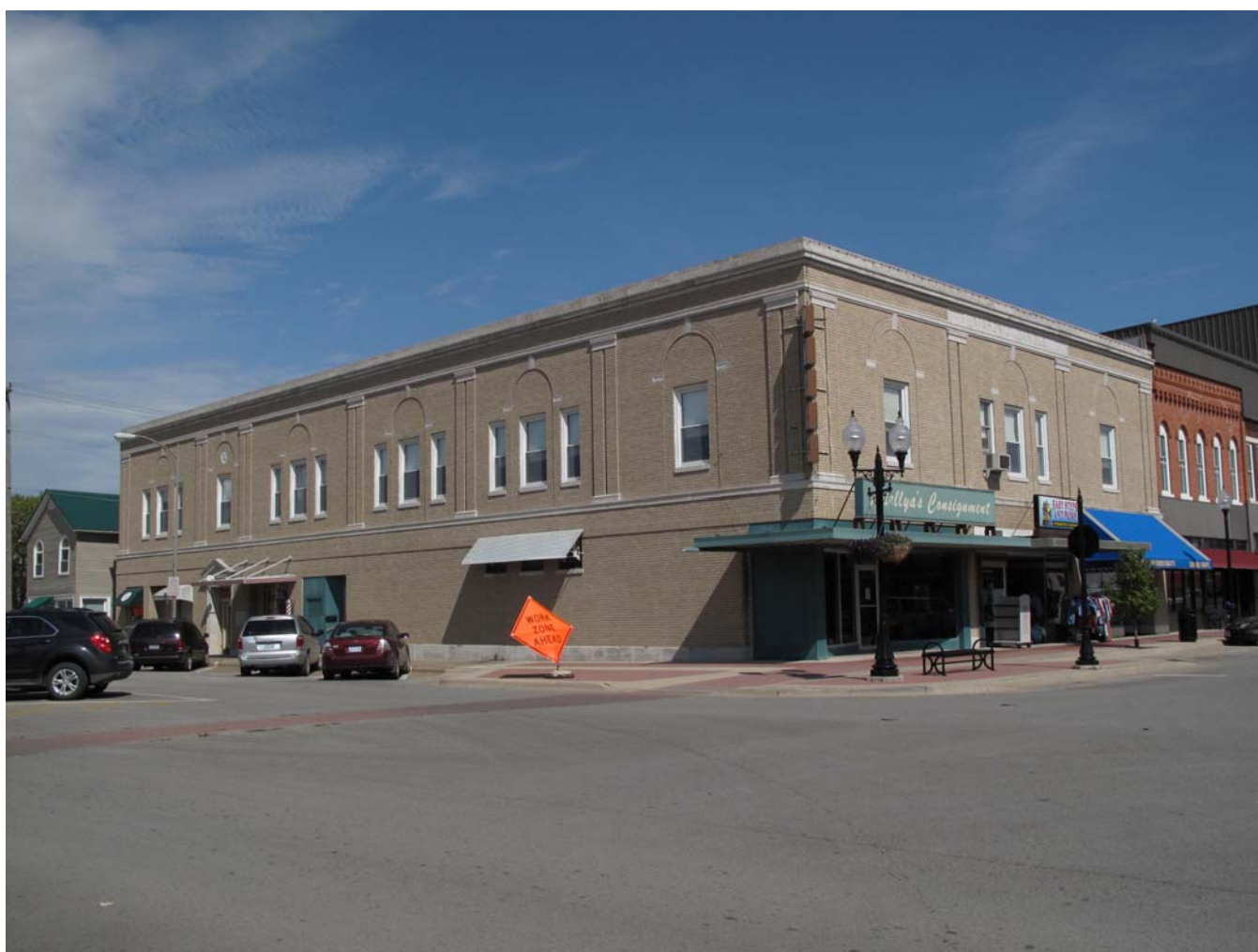
Photograph 92-00543-001 - West and south elevations, looking northeast (McCarley, September 20, 2011)
