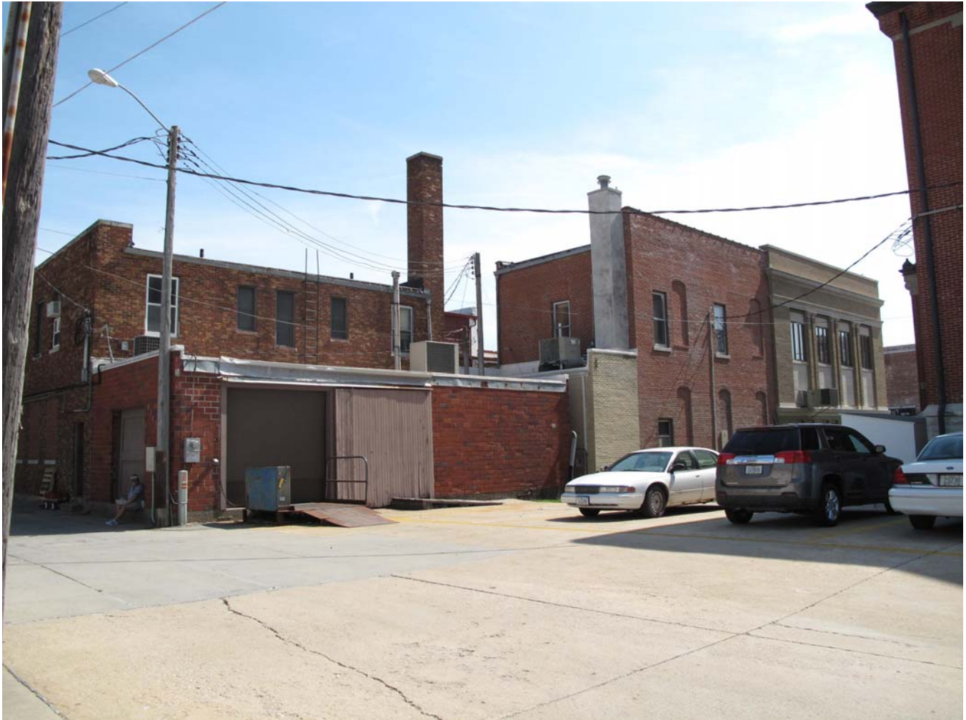
Photograph 92-00551-005 - West elevation, looking southeast (McCarley, September 20, 2011).
