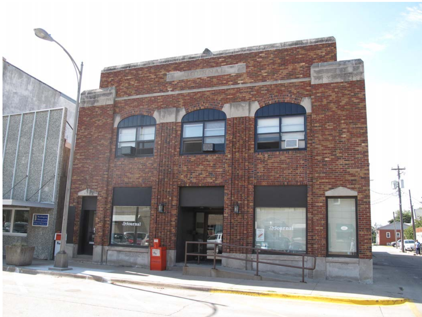
Photograph 92-00551-002 - East elevation, looking west (McCarley, September 20, 2011).
