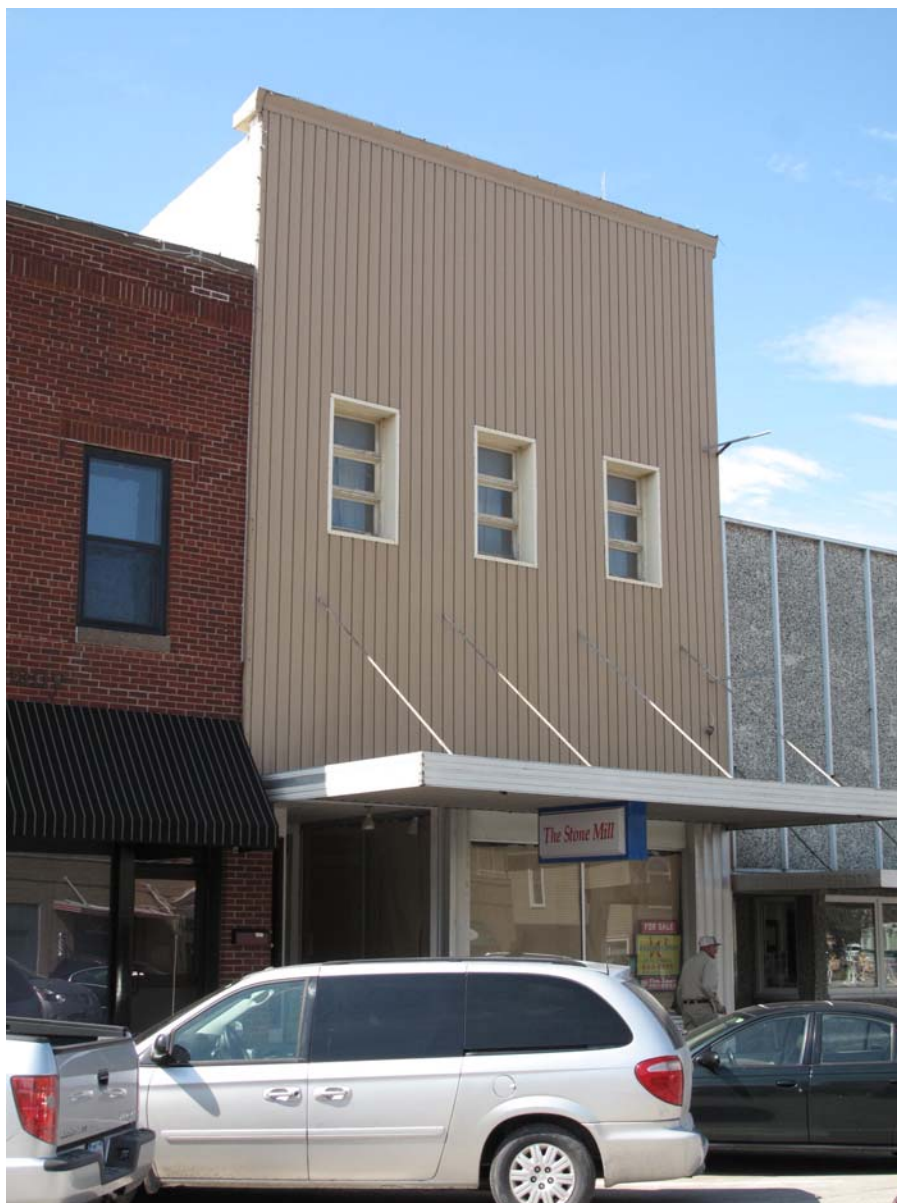
Photograph 92-00549-001 - East elevation, looking northwest (McCarley, September 20, 2011).
