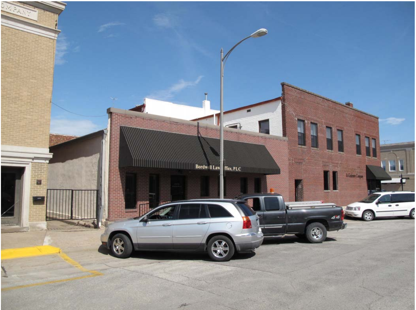
Photograph 92-00575-003 - West and south elevations, looking northeast (McCarley, September 20, 2011).
