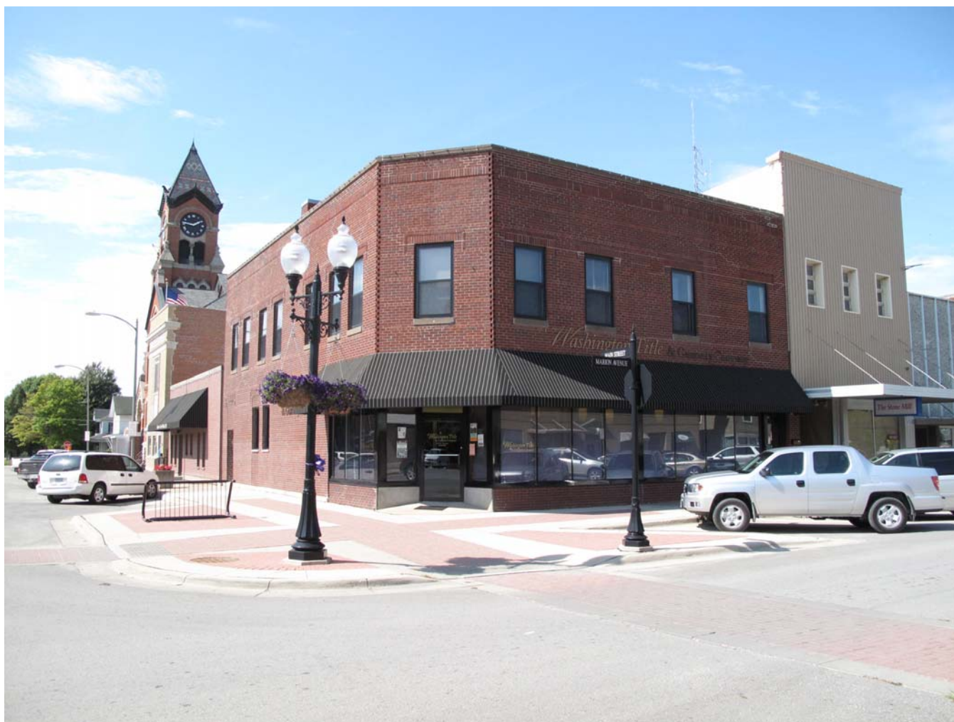
Photograph 92-00575-001 - South and east elevations, looking northwest (McCarley, September 20, 2011).
