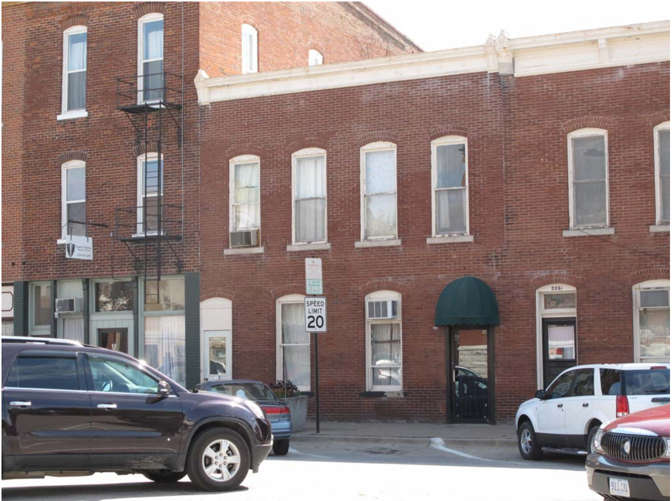
Photograph 92-00546-001 - Front (north) elevation of building, looking southeast (McCarley, September 20, 2011)
