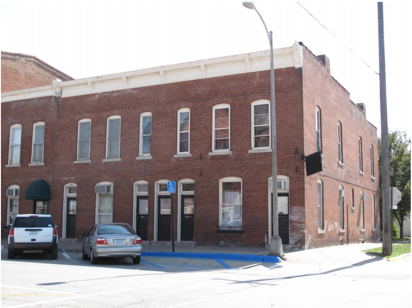
Photograph 92-00547-001 - Front (north) and west side elevations, looking southeast (McCarley, September 20, 2011).
