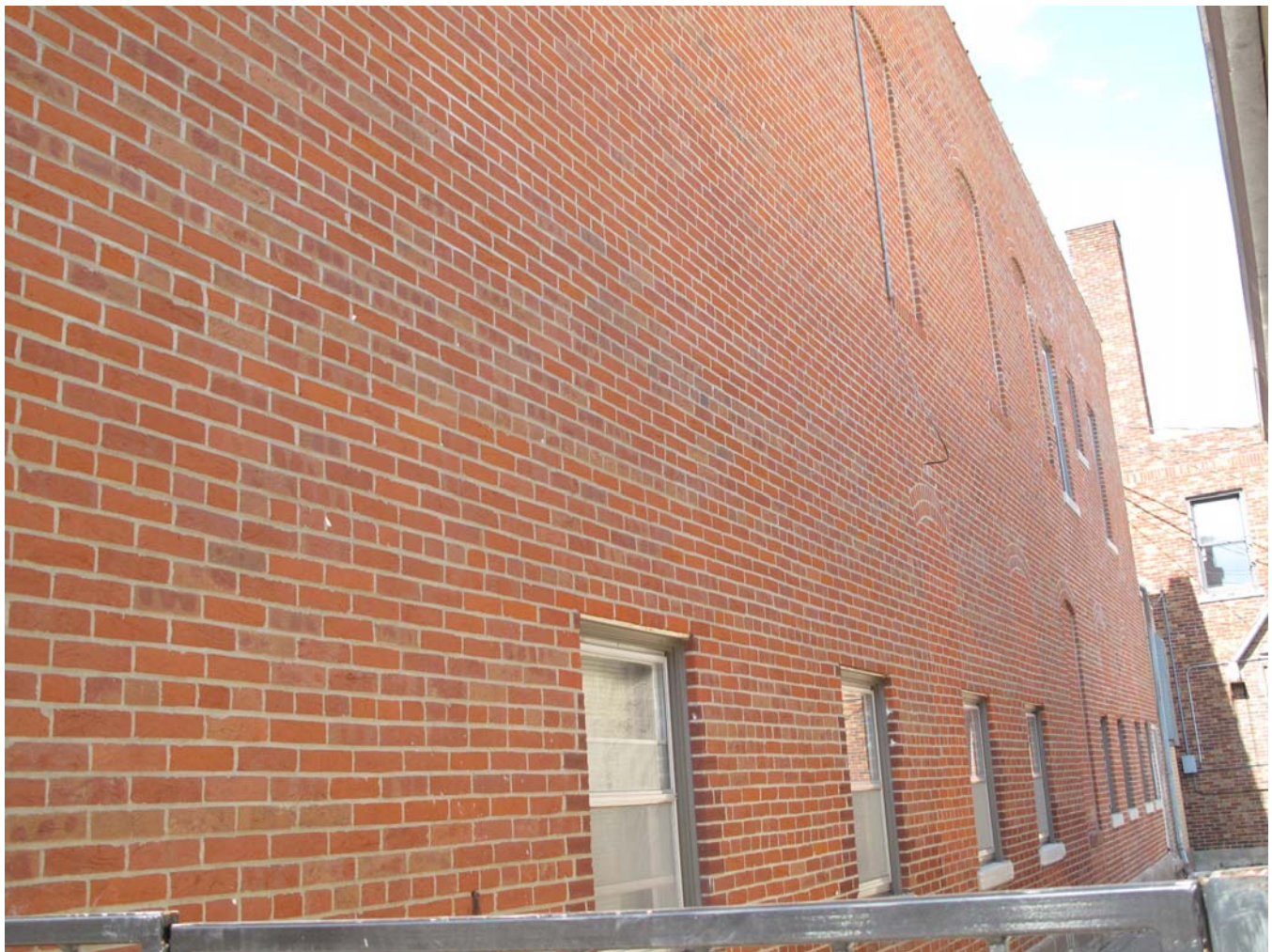
Photograph 92-00544-003 - East elevation, looking northwest (McCarley, September 20, 2011).
