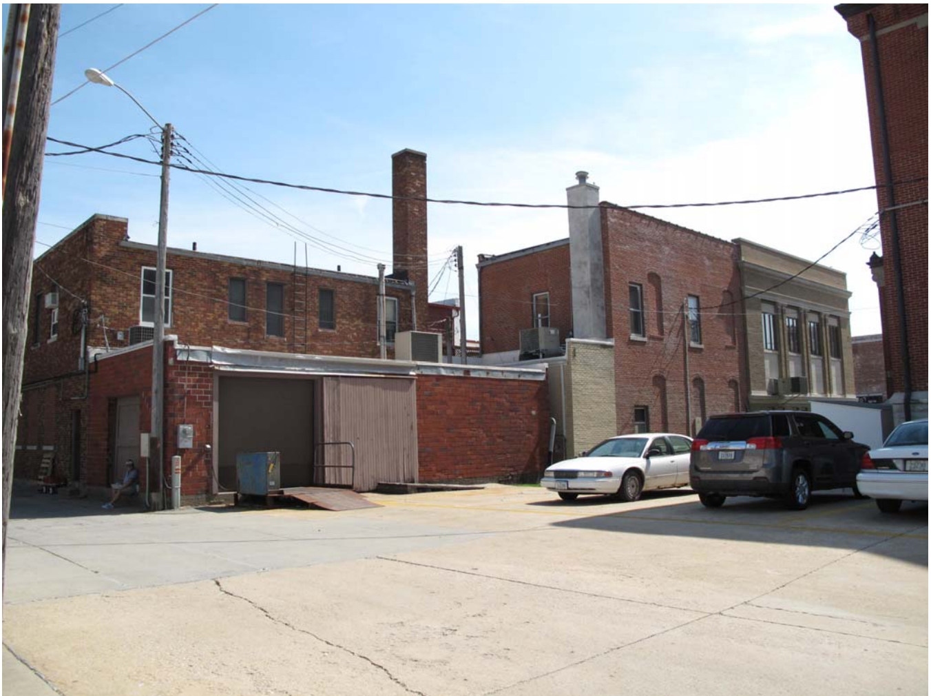
Photograph 92-00544-002 - Rear (north) and west elevations, looking southeast (McCarley, September 20, 2011).
