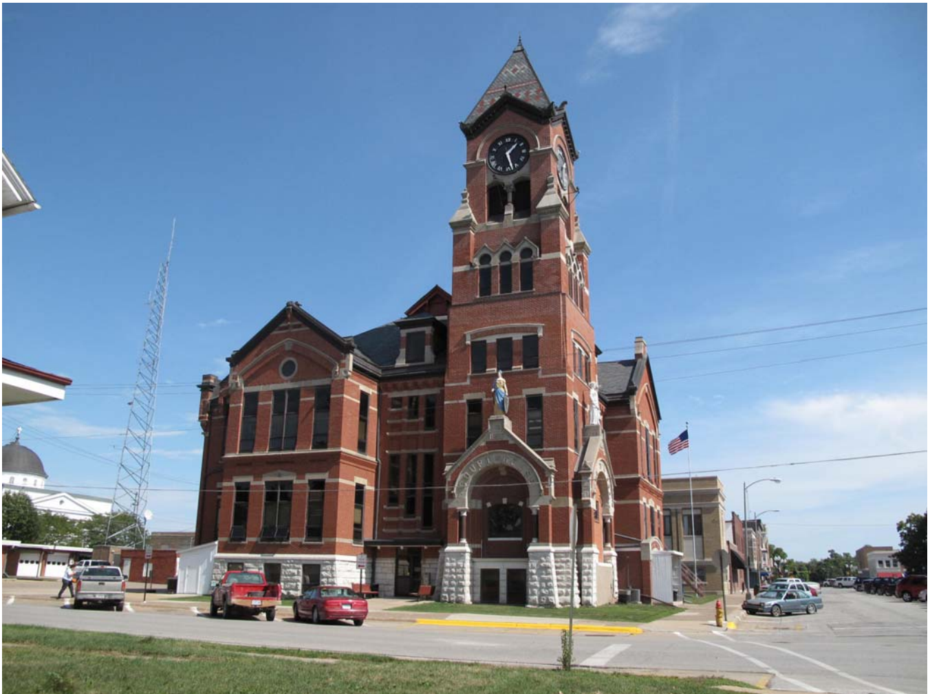
Photograph 92-00150-002 - Courthouse, looking east (McCarley, September 20, 2011)
