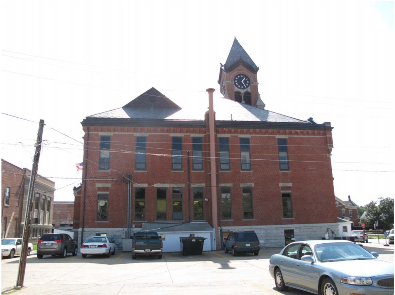
Photograph 92-00150-004 - Courthouse, looking south (McCarley, September 20, 2011)
