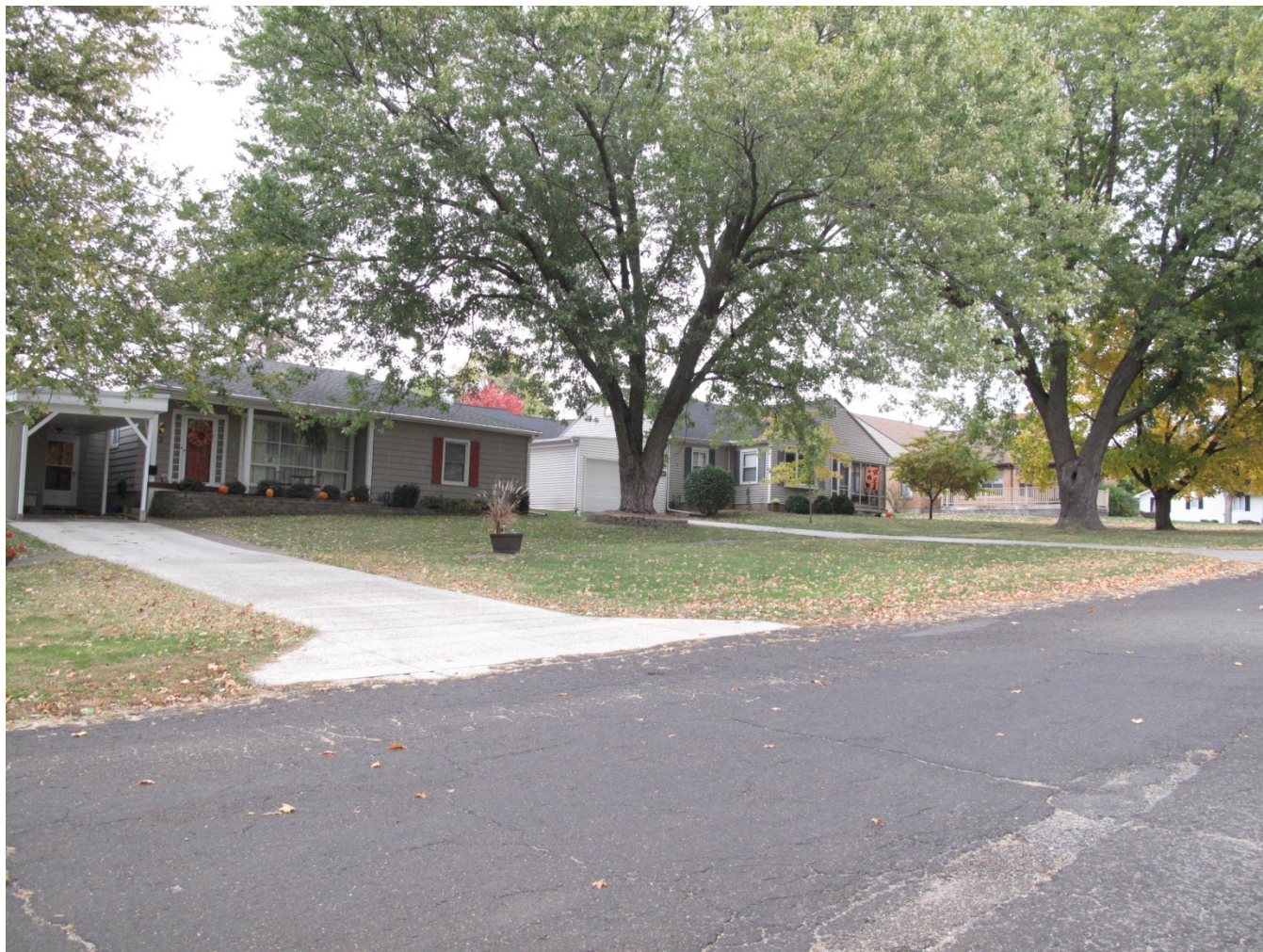
Photograph 92-00350-008 – 712-708-704 W. Washington Blvd (Map #85-84-83), looking northeast (October 2015)
