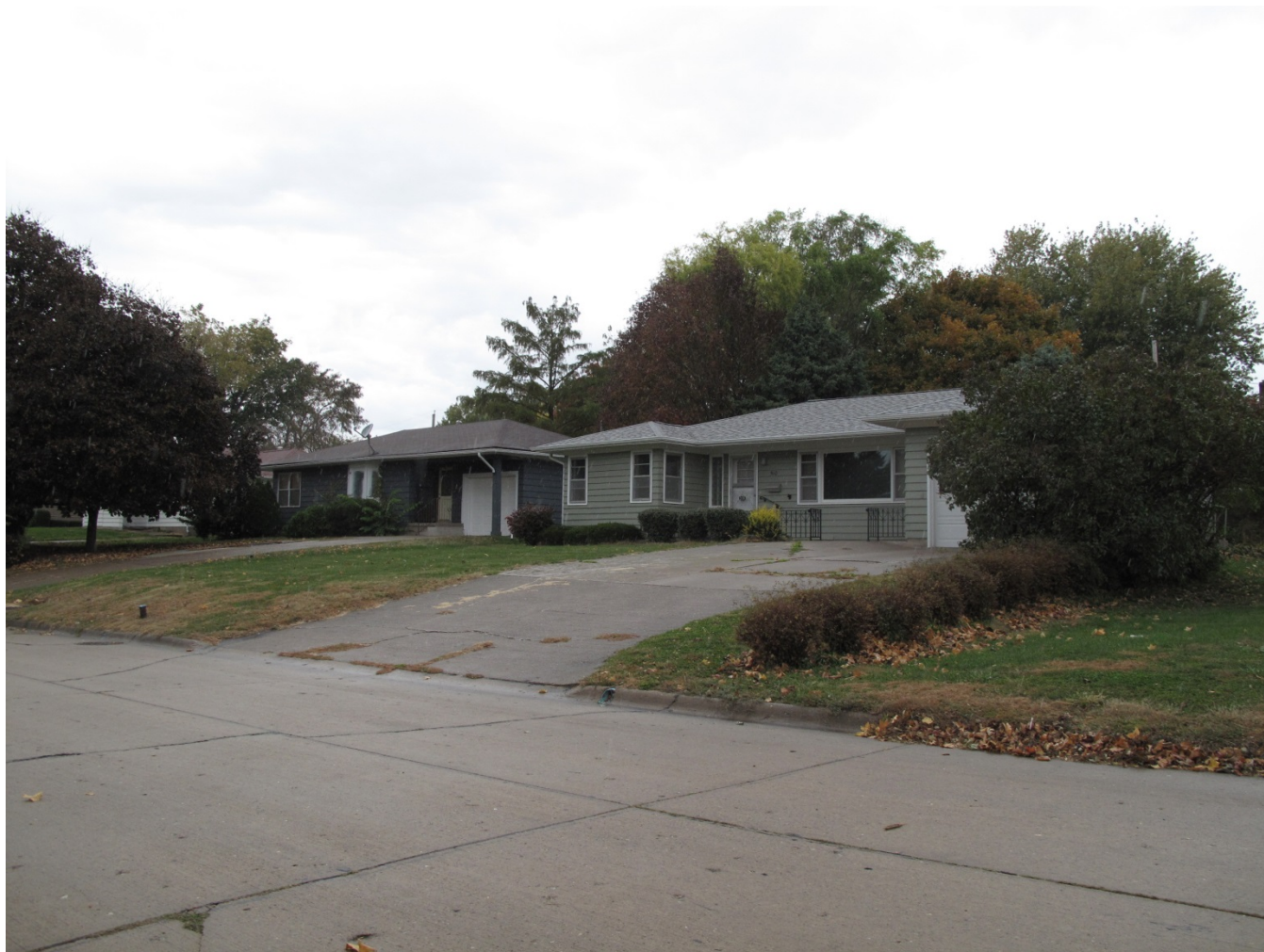
Photograph 92-00350-002 – 516-510 W. Jefferson (Map #26-25), looking northeast (October 2015)
